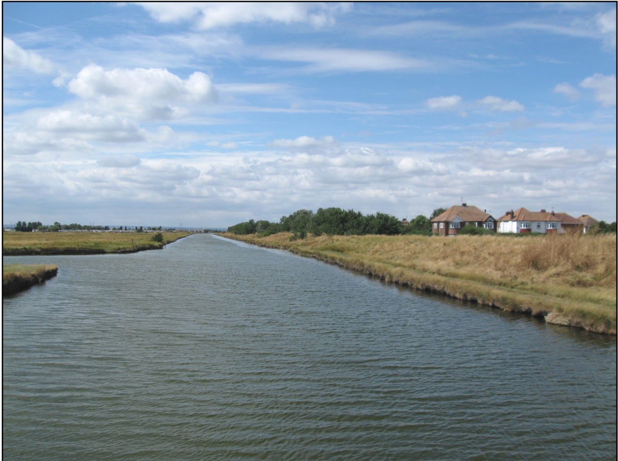
Queenborough Lines embankment shown on right-hand side of canal. Photograph taken August 2010.
